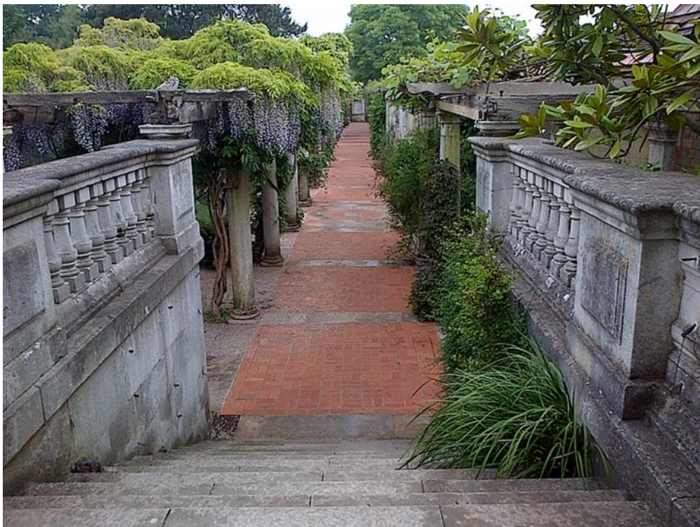
Section 2: general view showing renewed brick pavements.
