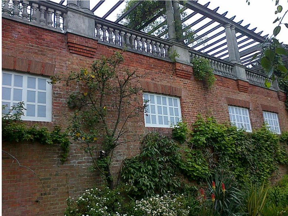
Section 2: The false windows after renovation in 2013.
